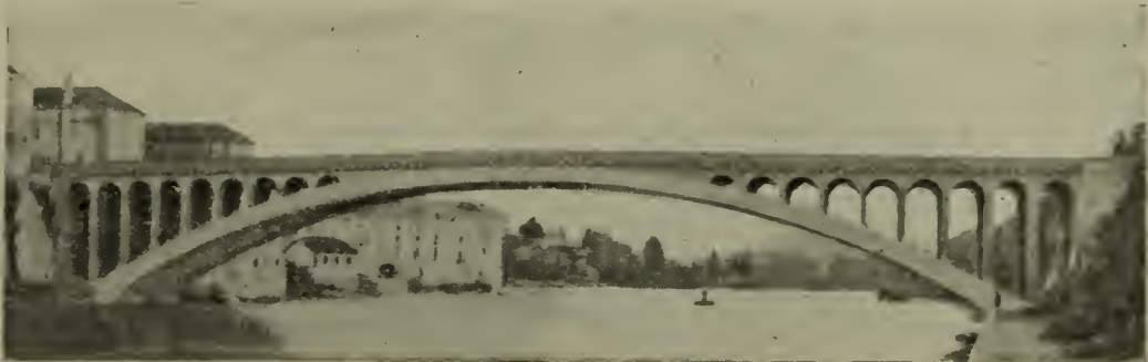
FIG. 1. THE VILLENEUVE BRIDGE.
